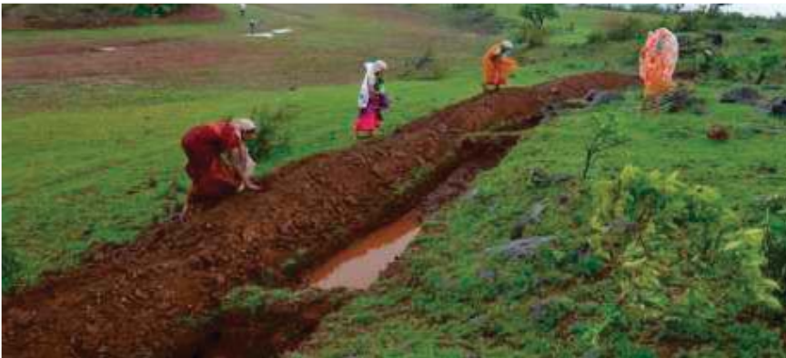
Construction of Water Absorption Trenches in Gondoshi
